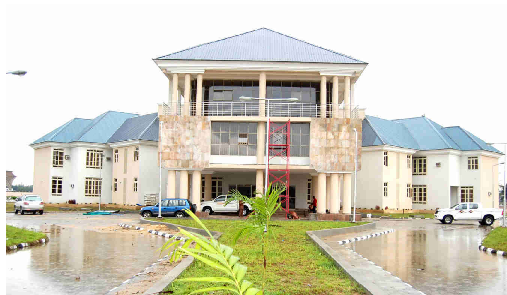
MULTI DOOR COURT HOUSE, YENAGOA
